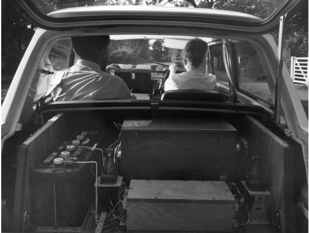
Figure 14: Instrumented car used by Dr Ivan Brown to measure drivers' spare mental capacity, c. 1965.
